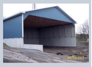
The salt shed project is going well and is on schedule. The roof and walls have been installed and the concrete floor will be poured the week of April 12th.
